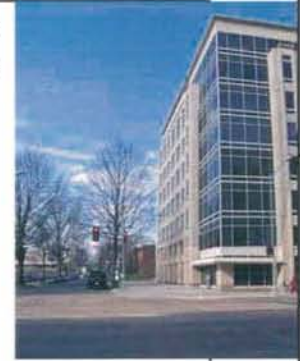
Looking north from the intersection of M Street, SE and 3rd Street, SE 300 M Street office building
